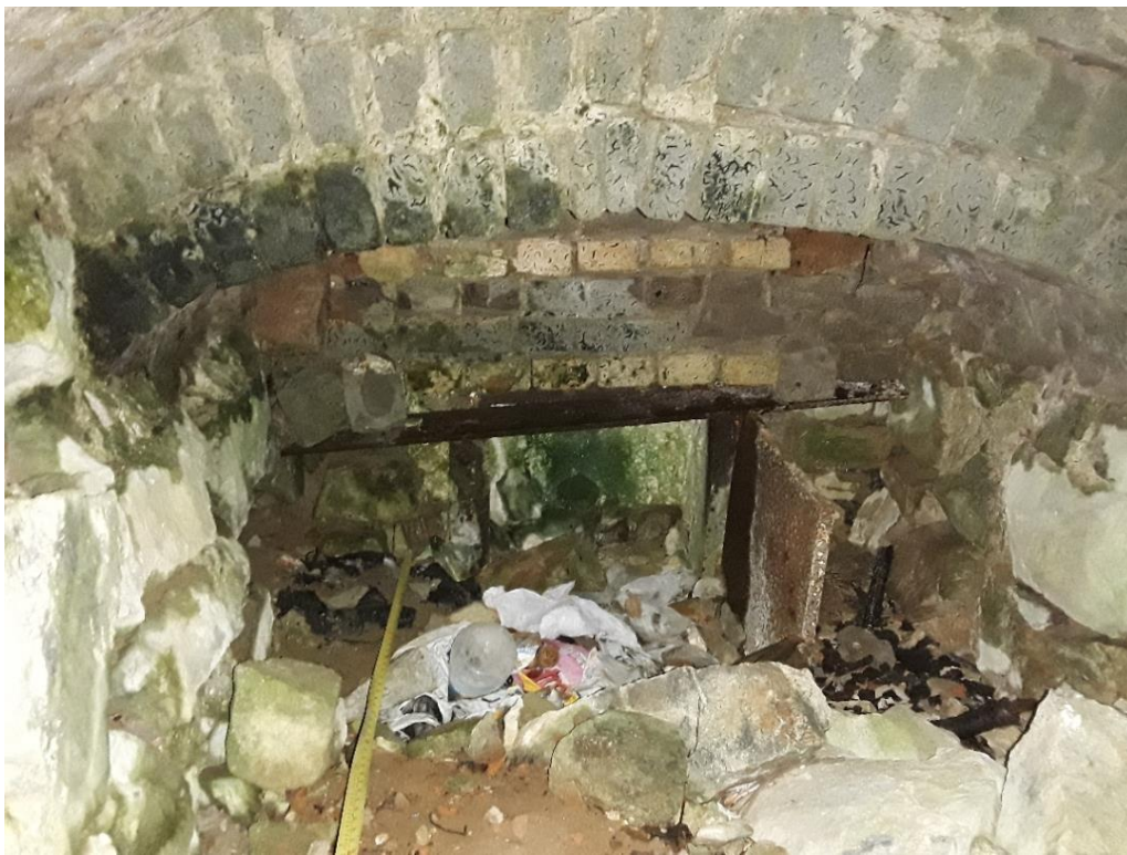
Figure 10. Inside of the drawhole chamber. The floor has been mostly filled with dirt, rubble and some garbage.
