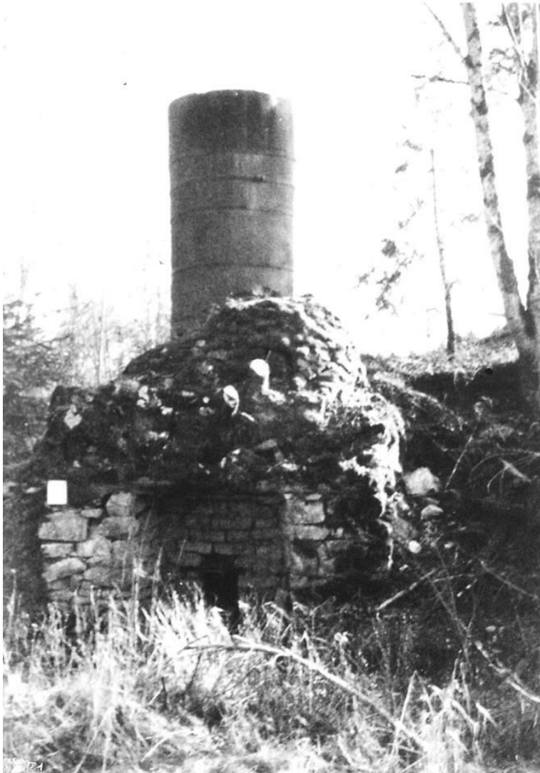
Figure 6. Kingzett Lake Lime Kiln, historic photograph (Shawnigan Lake Museum).
