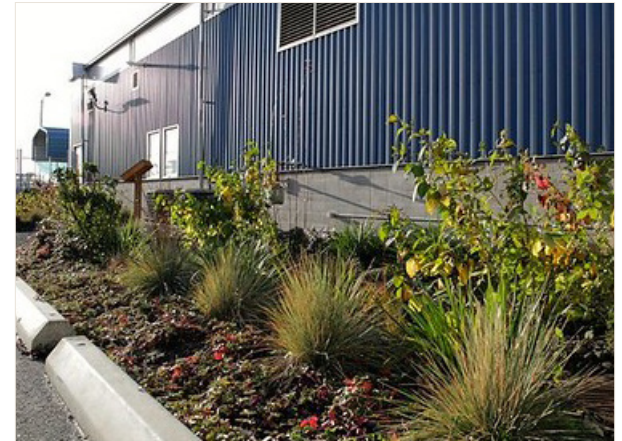
Bioswales reduce stormwater run-off.
