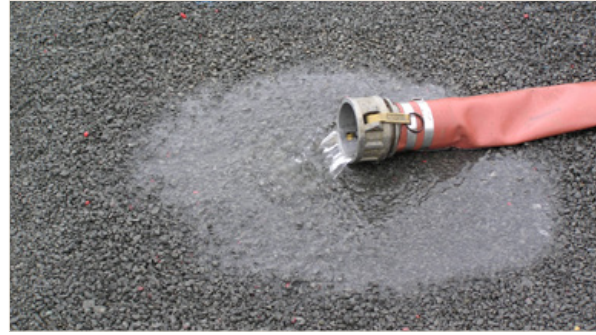
Porous asphalt paving reduces run-off in paving areas.
