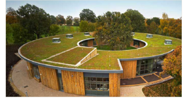
Green roofs store and utilize stormwater to reduce runoff from building sites.
