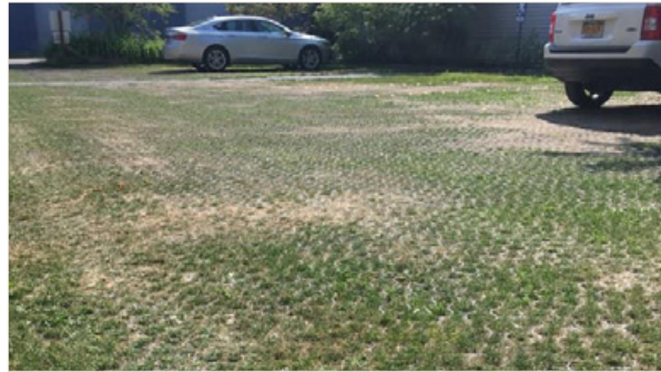
Structural grid paving reduces runoff in parking areas.
