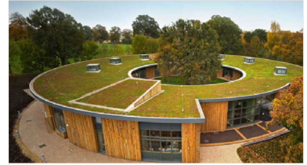
Green roofs store and utilize stormwater to reduce runoff from building sites.
