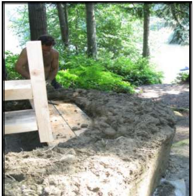
Gord Baird working on the Eagle Lake cob washroom
